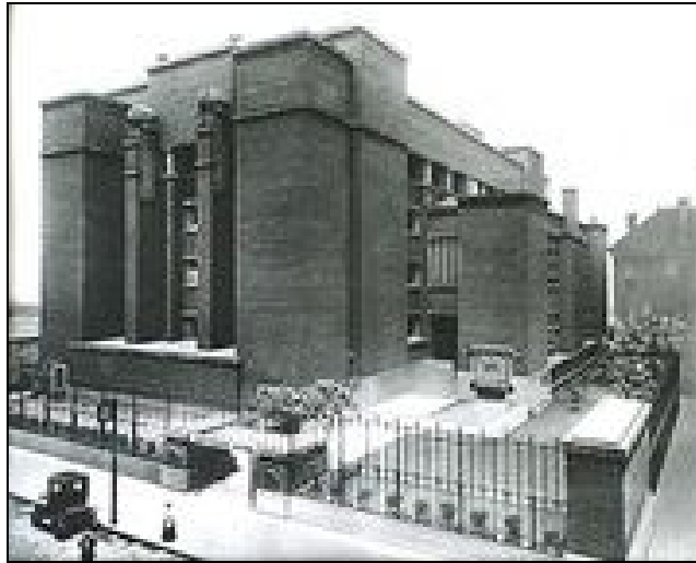
LARKIN ADMINISTRATION BUILDING
