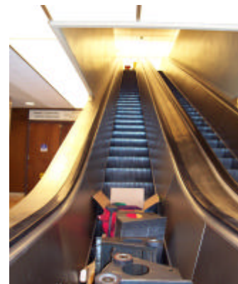
Pictured: Broken flange brackets required custom fabrication to repair/replace.
