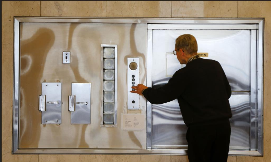
A librarian uses a book lift to transport a book from one floor to another. When customers aren't able to find a book on the shelves, a librarian sends a request to a page who finds the material in the stacks, which are on a floor not open to the public. Mark Mullette/Buffalo News
