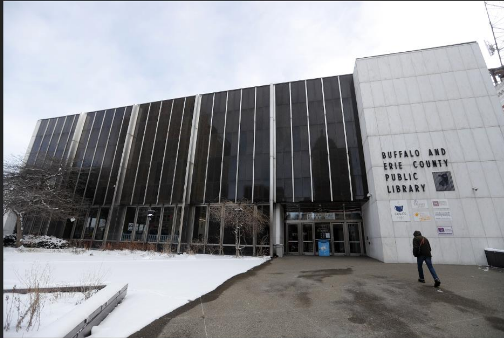
The concrete ramp in front of the library is heated by coils in the winter weather, so when it snows, the snow doesn't stick. Mark Mulville/Buffalo News
