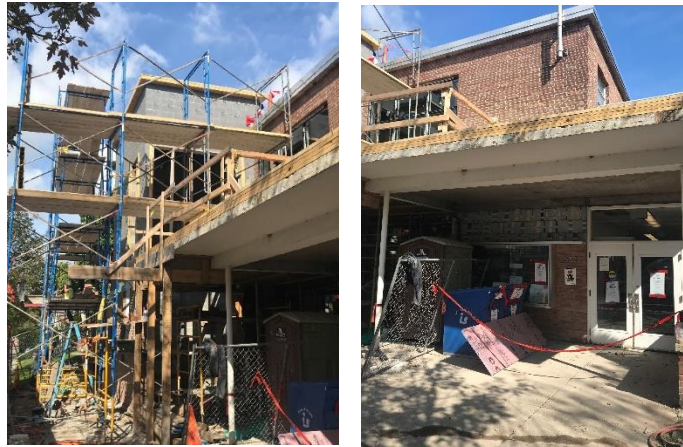
Crane Branch Library under construction
