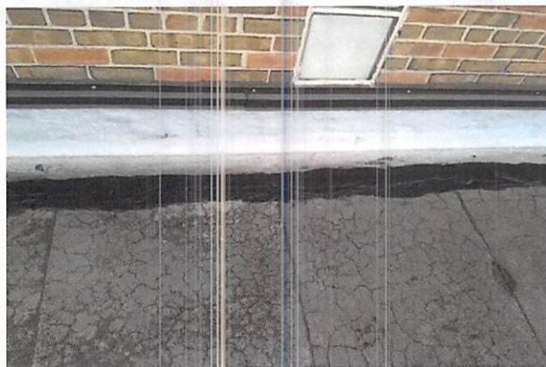
Reinforced exposed scrim.
