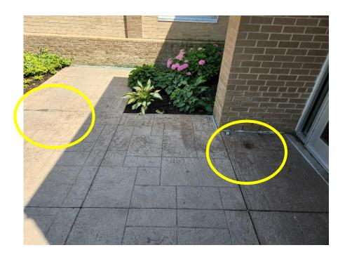
**Part 2:** cracked concrete located adjacent to the North entrance walkway, next to the employee entrance. Two slabs need to be renovated. The crack heaves in the winter and is a tripping hazard.
